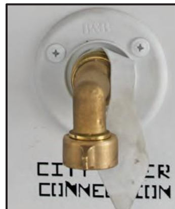
Figure 13-7: City Water Supply Connection
