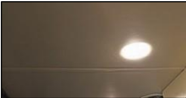
Figure 12-3: Typical Ceiling in the Allegro
