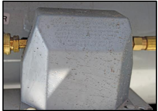
Figure 2-4: LP Gas Regulator
