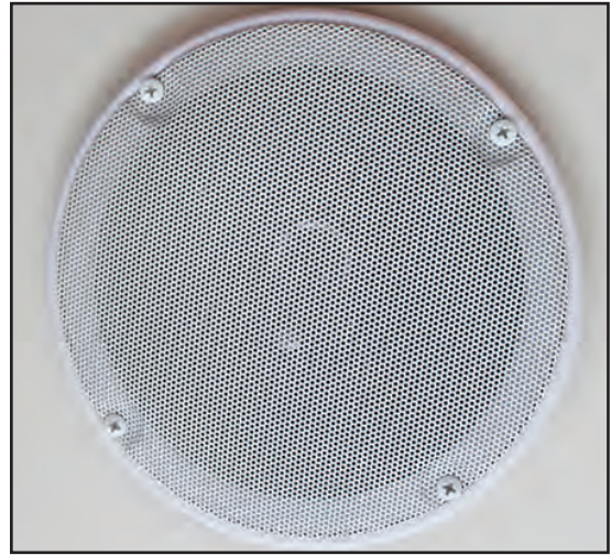
Figure 6-3: Overhead surround sound speaker
