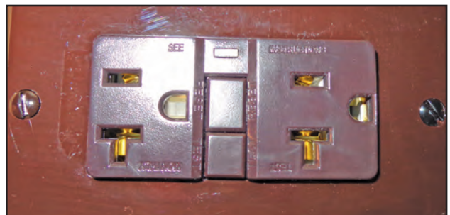
Figure 9-7: GFCI receptacle
