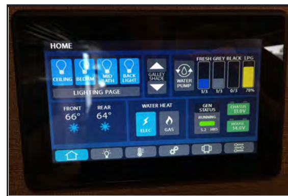
Figure 5-8: Water Heater Control Screen
