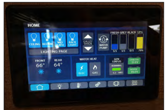
Figure 13-5: Water pump switch
