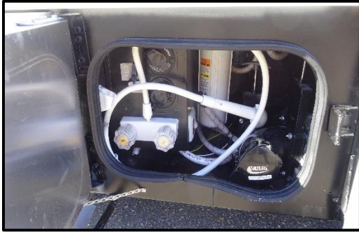
Figure 12-6: Motorhome Sewer Bay
