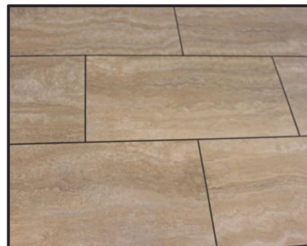
Figure 11-1: Typical Flooring in the MIDAS
