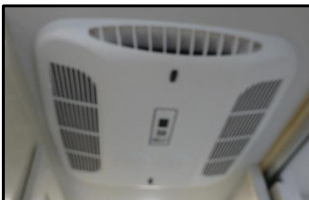
Figure 3-2: Outgoing/Return Air Vent
