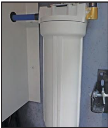
Figure 12-7: Water Filter
