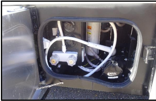
Figure 12-6: Motorhome Sewer Bay
