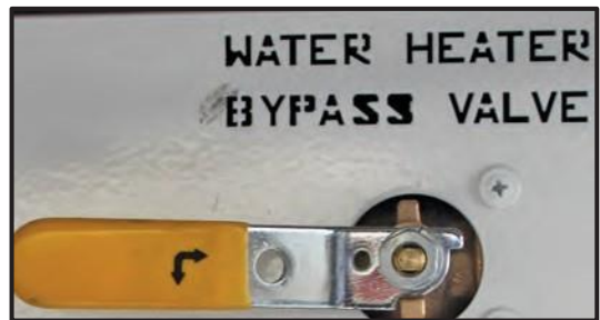
Figure 13-9: Water Heater Bypass System
