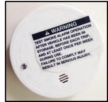
Figure 2-7: Smoke Detector
