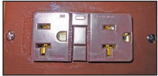
Figure 9-6: GFCI Receptacle
