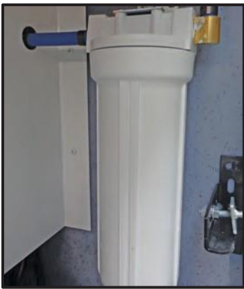
Figure 13-8: Water Filter
