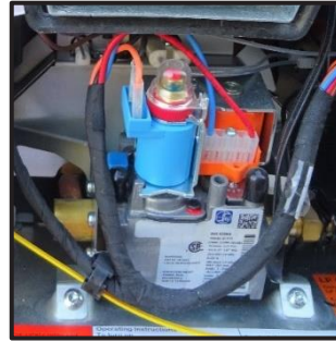
Figure 5-9: Water Heater Relief Valve
