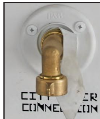
Figure 13-7: City Water Supply Connection
