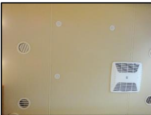
Figure 12-3: Typical Ceiling in the Allegro RED
