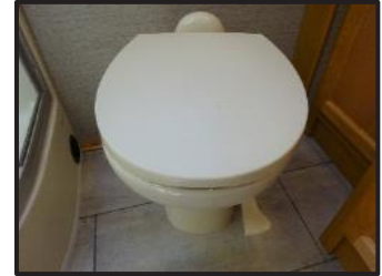
Figure 13-10: Toilet Pedal Flush Lever
