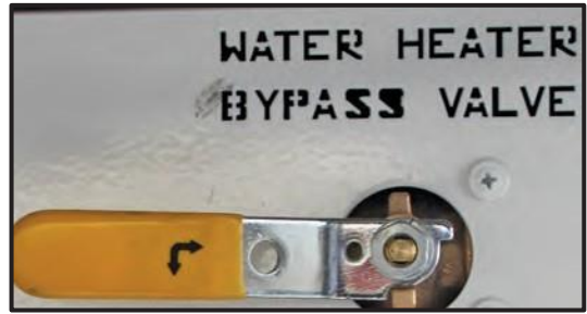
Figure 13-9: Water Heater Bypass System
