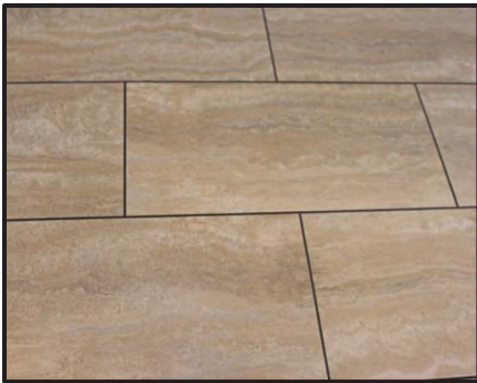
Figure 12-2: Typical Flooring in the Allegro RED 340
