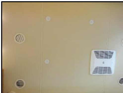
Figure 12-3: Typical Ceiling in the Allegro RED
