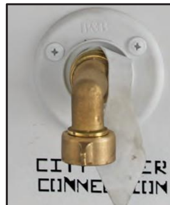
Figure 13-7: City Water Supply Connection
