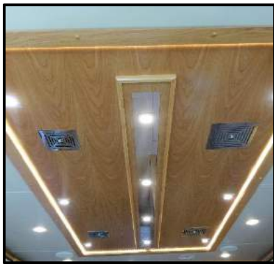
Figure 12-3: Typical Ceiling in the Allegro RED
