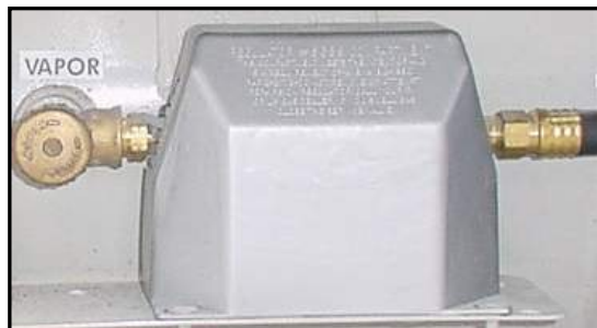
Figure 3-5. LP Gas Regulator
