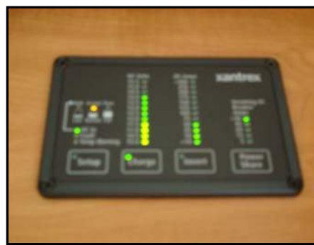
Figure 7-13. Inverter Control Panel
