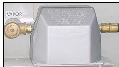
Figure 2-6. LP Gas Regulator
