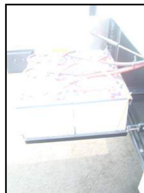
Figure 7-6. Batteries on Slide Tray
