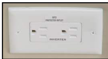
Figure 7-11. GFCI Receptacle
