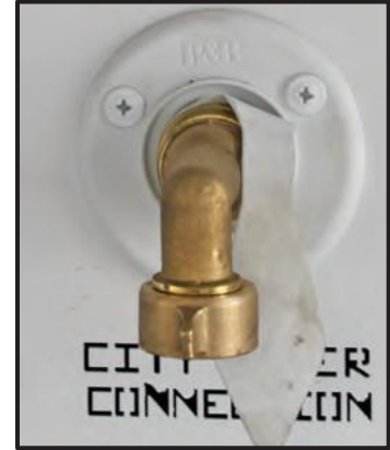
Figure 13-7: City Water Supply Connection
