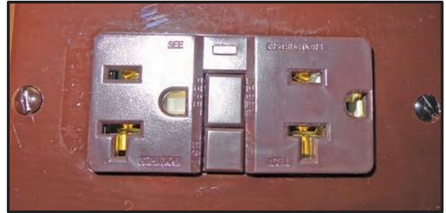
Figure 9-5: GFCI Receptacle
