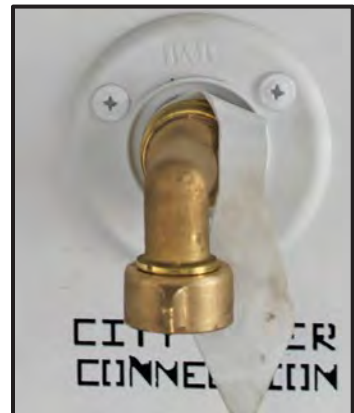
Figure 13-7: City Water Supply Connection
