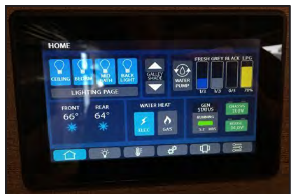
Figure 5-9: Water Heater Control Screen
