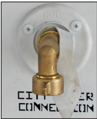
Figure 13-6: City water supply connection
