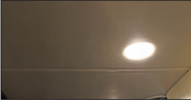
Figure 12-3: Typical ceiling in the Allegro RED
