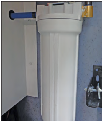
Figure 13-8: Water filter
