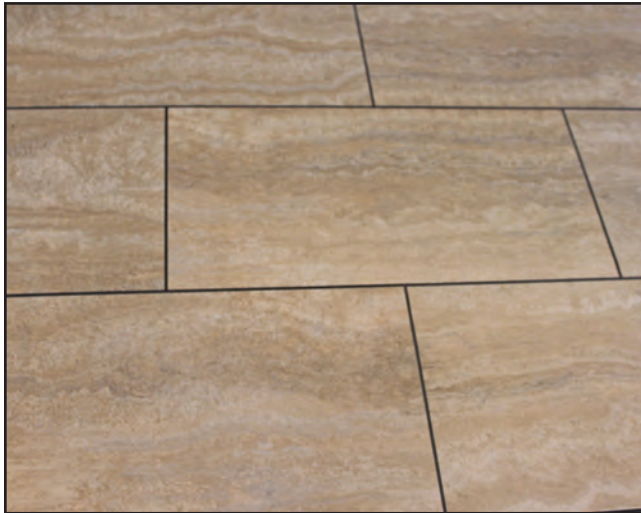
Figure 12-2: Typical flooring in the Allegro RED
