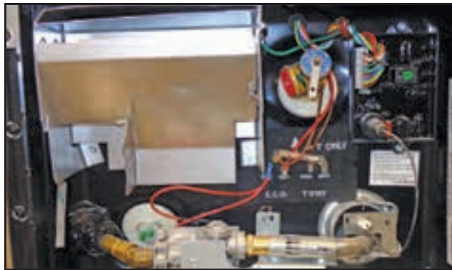
Figure 5-8: Water heater
