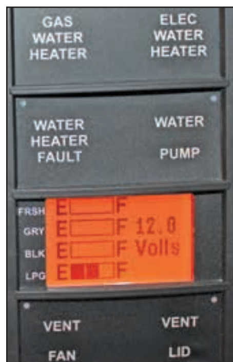
Figure 5-7: Water heater switches
