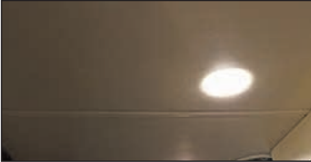
Figure 12-3: Typical ceiling in the Allegro RED
