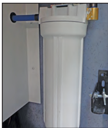
Figure 13-8: Water filter
