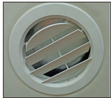
Figure 3-4: Round air vent
