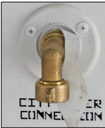
Figure 13-6: City water supply connection
