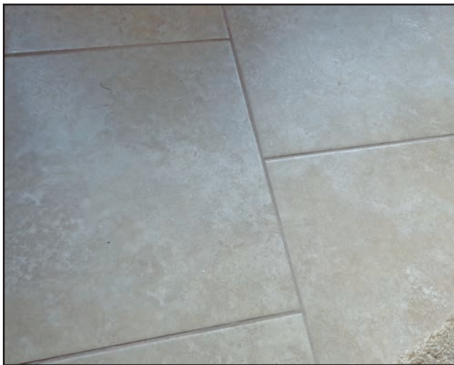
Figure 12-2: Typical flooring in the Allegro RED
