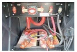
Figure 7-5. 12 VDC Battery System
