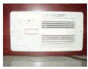
Figure 4-22. Carbon Monoxide/LP Gas Detector
