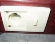
Figure 13-13. Vacuum Hose Coupling
