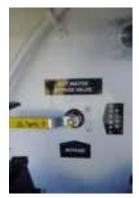
Figure 11-9. Water Heater Bypass System
