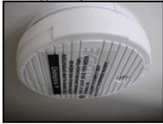
Figure 13-20. Smoke Detector
