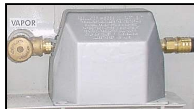
Figure 2-6. LP Gas Regulator
