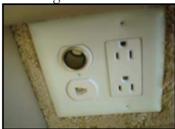
Figure 7-9. 120 VAC Receptacle
