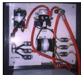
Figure 7-14. Circuit Breakers
