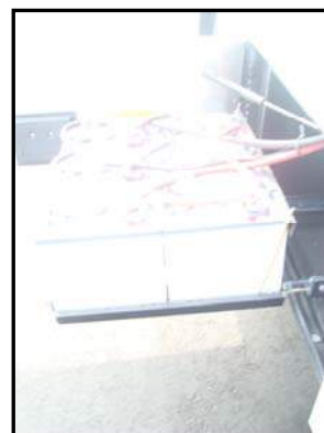
Figure 7-6. Batteries on Slide Tray
