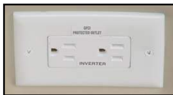
Figure 7-11. GFCI Receptacle
