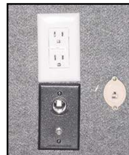
Figure 7-10. 12 VDC Receptacle (black)
