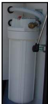
Figure 11-8. Water Filter
