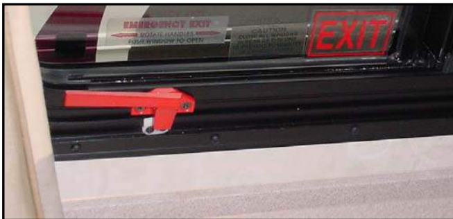
Figure 13-2. Bedroom Emergency Exit Window
