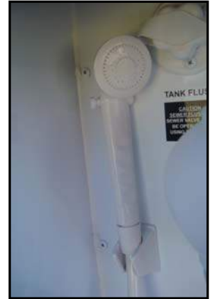
Figure 11-12. Exterior Shower and Exterior Light
