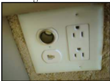
Figure 7-9. 120 VAC Receptacle
