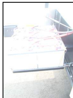
Figure 7-6. Batteries on Slide Tray
