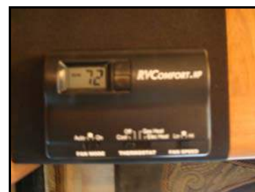
Figure 3-3. Thermostat
