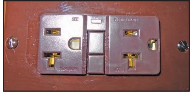
Figure 9-5: GFCI Receptacle
