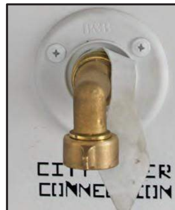
Figure 13-7: City Water Supply Connection
