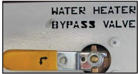
Figure 13-9: Water Heater Bypass System
