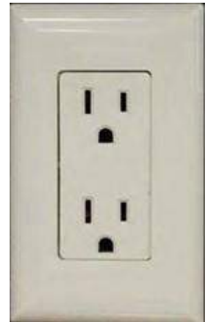
Figure 9-5: 120 VAC Receptacle
