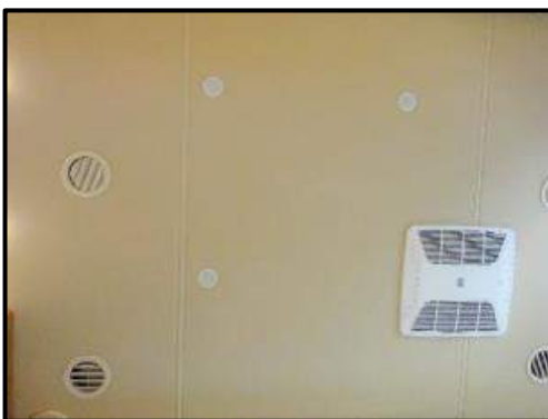
Figure 12-3: Typical Ceiling in the Allegro RED
