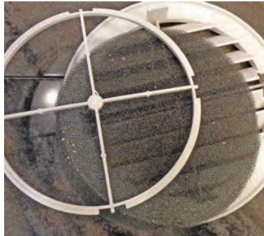
Figure 3-3: Round Vent Filter
