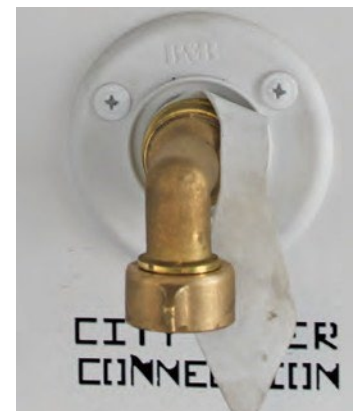
Figure 13-9: City Water Supply Connection
