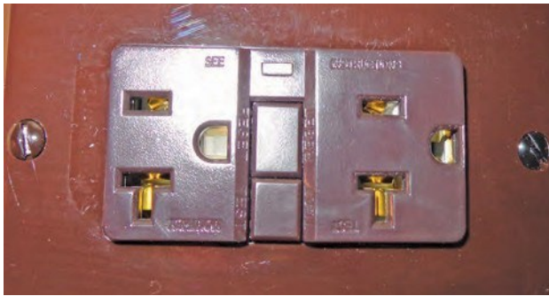
Figure 9-8: GFCI Receptacle
