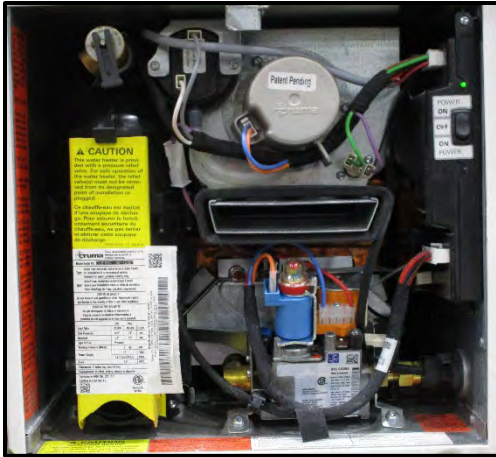
Figure 5-7: Water Heater
