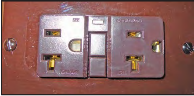
Figure 9-8: GFCI Receptacle
