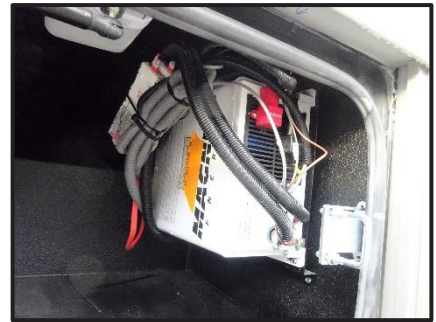
Figure 9-8: Converter/Inverter
