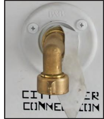
Figure 13-7: City Water Supply Connection
