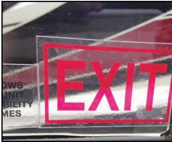
Figure 2-7: Emergency Exit Window
