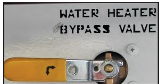
Figure 13-9: Water Heater Bypass System
