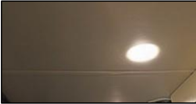
Figure 12-3: Typical Ceiling in the Allegro
