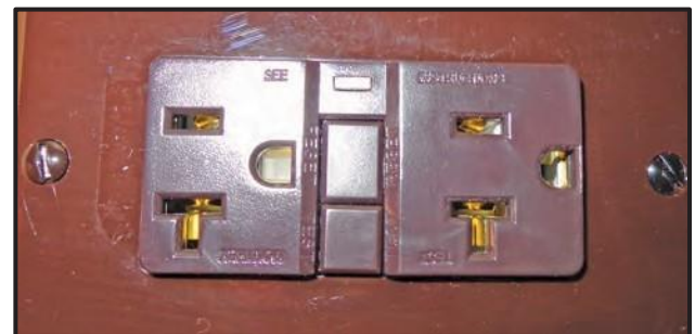
Figure 9-7: GFCI Receptacle
