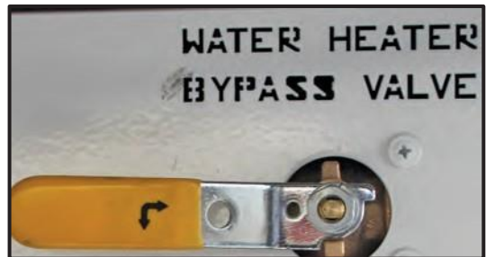
Figure 13-9: Water Heater Bypass System
