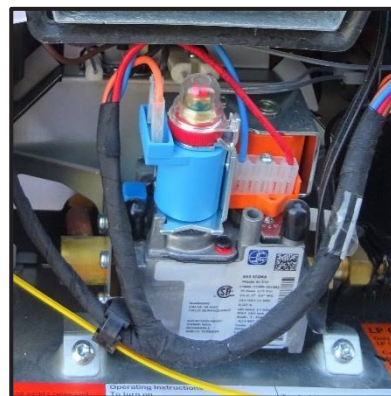
Figure 5-9: Water Heater Relief Valve
