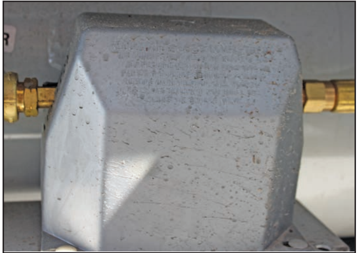
Figure 2-4: LP Gas Regulator
