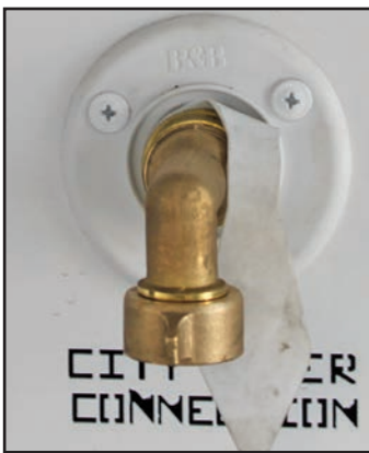
Figure 13-6: City water supply connection
