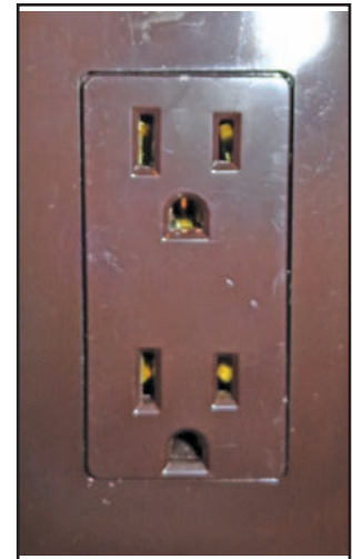
Figure 9-5: 120 VAC receptacle
