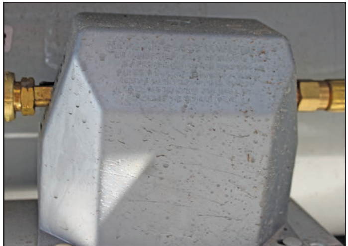
Figure 4-2: LP Gas Regulator
