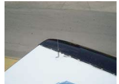
Figure 4-14. CB Antenna Installation
