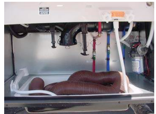
Figure 11-10. Wastewater Drain Hose and Connection in Sanitation Compartment
