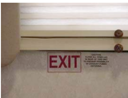
Figure 2-7. Emergency Exit Window
