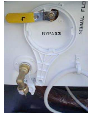
Figure 11-8. Water Heater Bypass System
