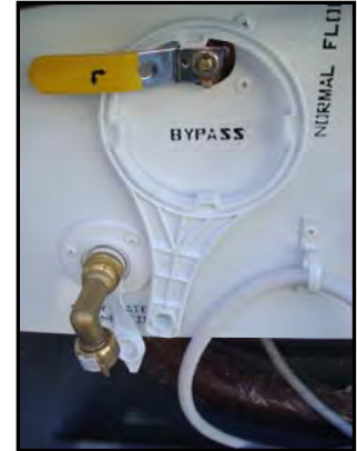
Figure 11-8. Water Heater Bypass System
