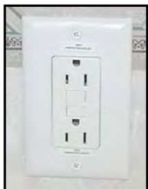
Figure 7-7. GFCI Receptacle
