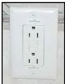
Figure 7-7. GFCI Receptacle
