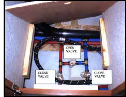
Figure 11-8. Water Heater Bypass System
