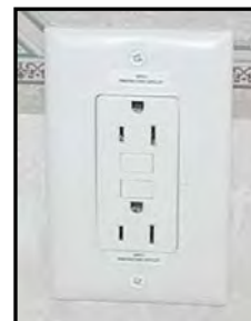
Figure 7-5. Typical AC Receptacle
