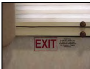
Figure 13-2. Emergency Exit Window
