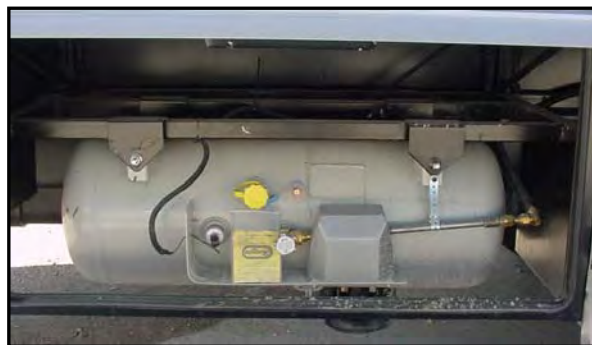
Figure 2-4. Liquid Propane Tank
