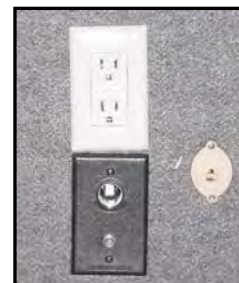
Figure 7-6. Typical 12VDC Receptacle (Bottom)
