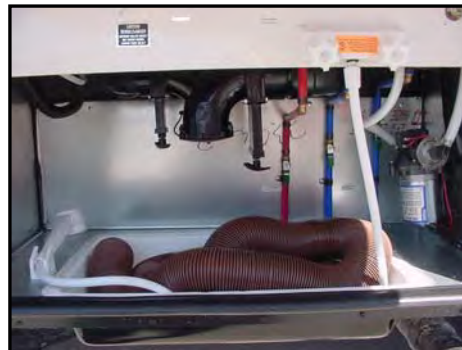
Figure 11-11. Exterior Shower in Outside Sanitation Compartment
