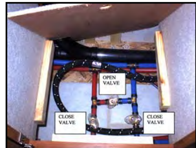
Figure 11-8. Water Heater Bypass System
