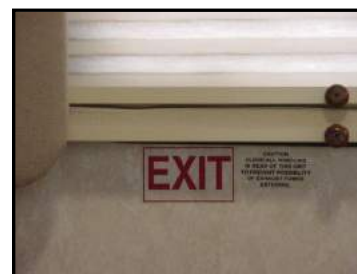
Figure 2-7. Emergency Exit Window
