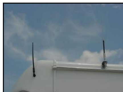
Figure 4-14. CB Antenna Installation
