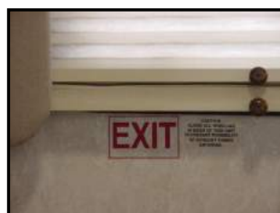
Figure 13-2. Emergency Exit Window
