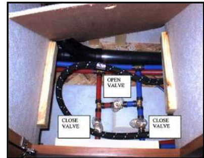
Figure 11-7. Water Heater Bypass System
