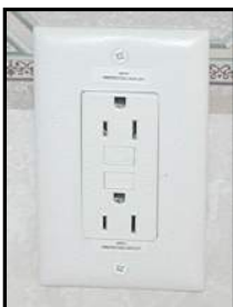
Figure 7-7. GFCI Receptacle
