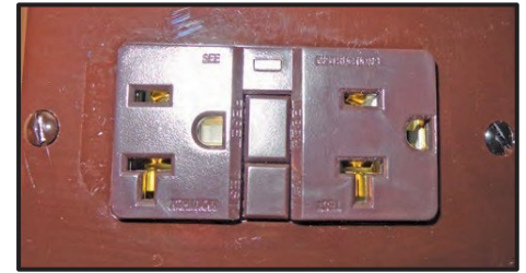
Figure 9-18: GFCI Receptacle
