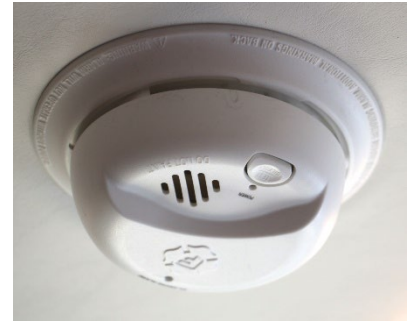
Figure 2-4: Smoke Detector
