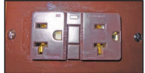
Figure 9-18: GFCI Receptacle
