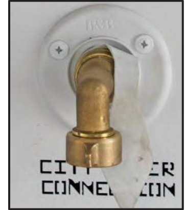
Figure 13-9: City Water Supply Connection
