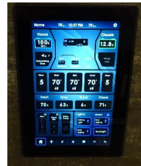
Figure 0-2: Home Screen for the Spyder Controls System
