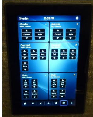
Figure 0-11: Day/Night Window Shade Control
