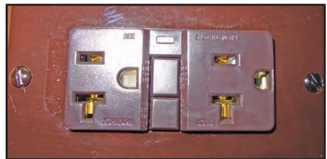
Figure 0-9: GFCI Receptacle
