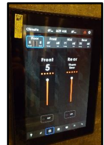
Figure 4-7: Heat Pump Controls
