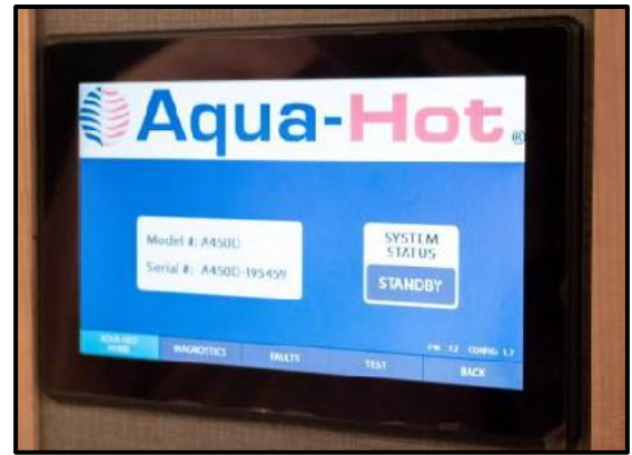
Figure 4-1: Aqua-Hot Heating System Control Screen
