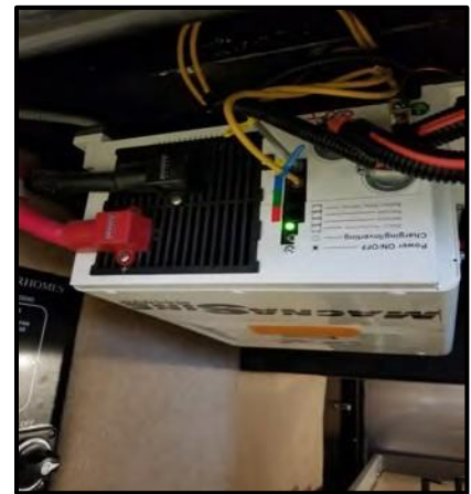
Figure 9-7: Converter/Inverter
