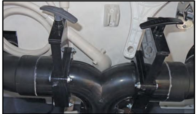
Figure 13-14: Sanitation Coupling
