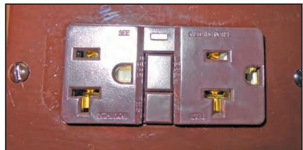
Figure 9-12: GFCI receptacle
