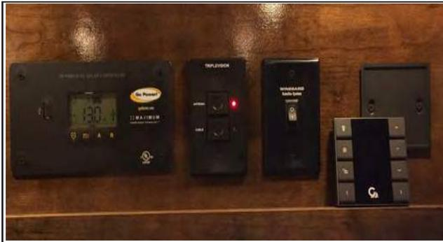
Figure 14-2: Removable Awning Remote Switch location
