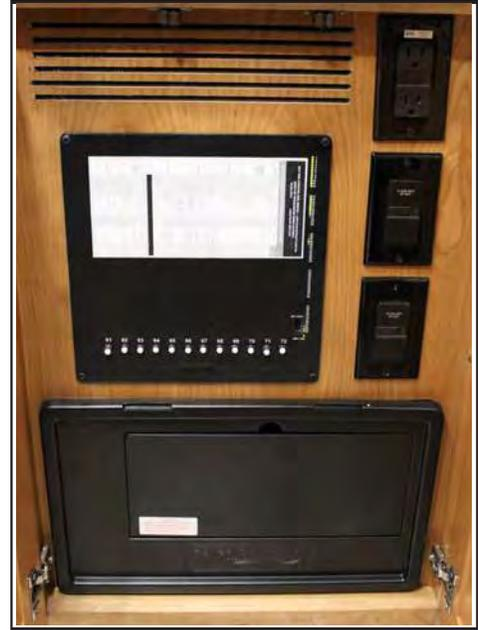
Figure 9-16: Circuit breakers
