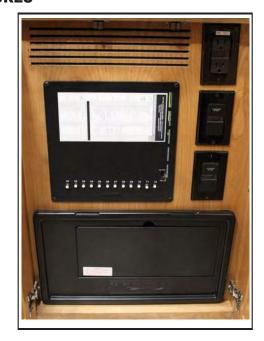
Figure 9-16: Circuit breakers
