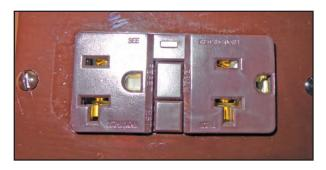
Figure 9-12: GFCI receptacle
