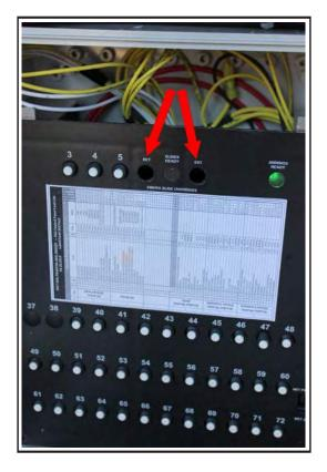
Figure 10-4: Location of Slide-out room control override
