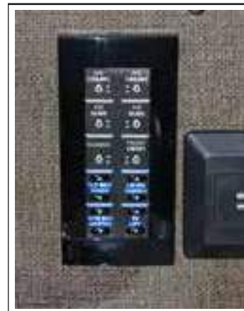
Figure 11-6 : Day/night window shade control
