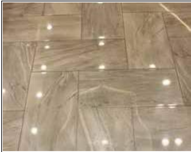
Figure 11-2: Typical flooring in the Allegro Bus
