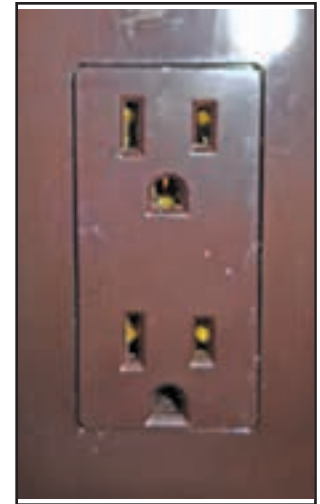
Figure 9-5: 120 VAC receptacle
