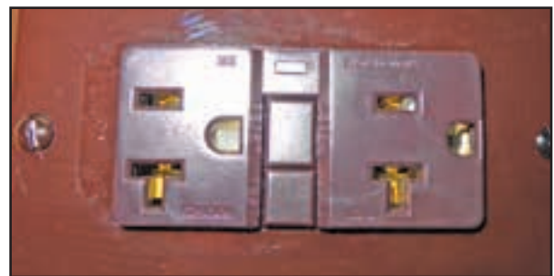
Figure 8-11: GFCI receptacle
