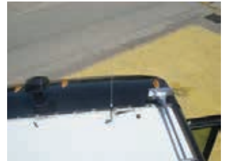
Figure 4-17. CB Antenna Installation
