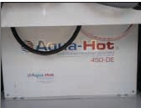
Figure 3-2. Hydraulic Heating System
