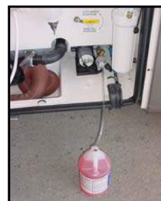
Figure 13-16. Winterizing the Water System
