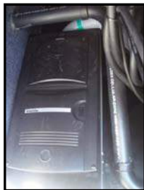
Figure 13-10. Vacuum Cleaner System
