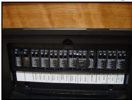
Figure 7-19. Resettable Circuit Breakers
