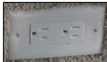
Figure 7-11. 120 VAC Outlets
