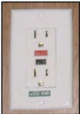
Figure 7-14. Ground-Fault Circuit Interrupter (GFCI)
