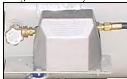
Figure 3-8. LP Gas Regulator
