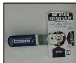
Figure 11-10. Water Heater Bypass
