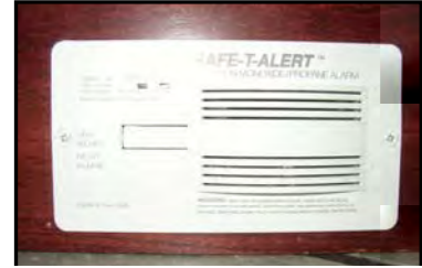
Figure 3-9. CO/LP Gas Detector
