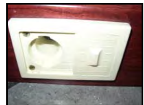
Figure 13-9. Vacuum Hose Coupling
