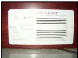
Figure 4-23. Carbon Monoxide/LP Gas Detector
