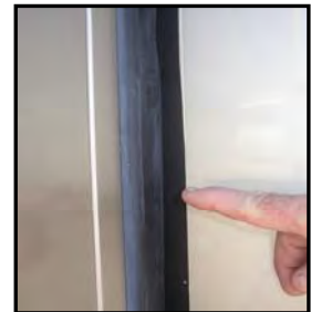
Figure 13-6. Inspecting Slide Out Gasket
