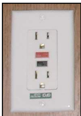
Figure 7-13. Ground-Fault Circuit Interrupter (GFCI)
