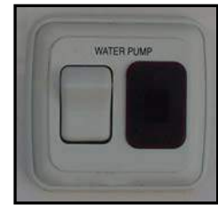
Figure 11-6. Water Pump Switch
