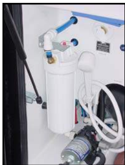
Figure 11-9. Water Filter
