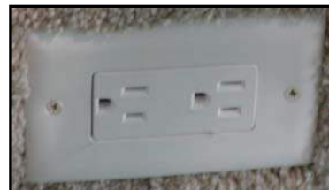
Figure 7-11. 120 VAC Outlets
