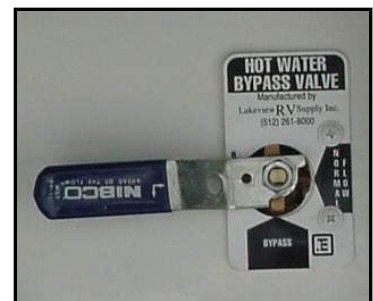
Figure 11-10. Water Heater Bypass
