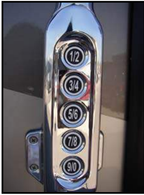
Figure 13-8. Detail of Keyless Lock
