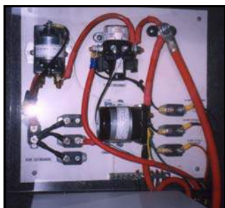
Figure 7-16. Resettable Circuit Breakers
