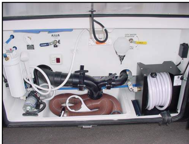
Figure 11-13. Sanitation Compartment Containing Holding Tank Drains and Flexible Drain Hose
