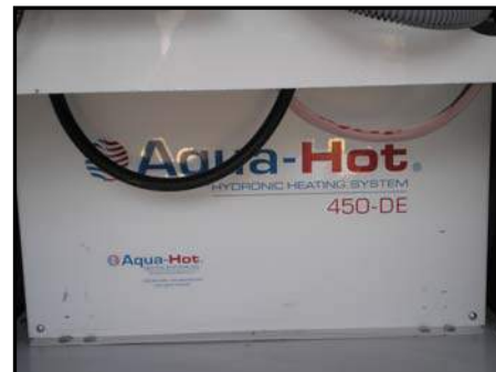
Figure 11-16. Hydraunic Heating System
