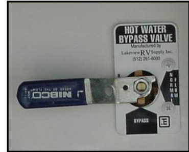
Figure 11-11. Water Heater Bypass
