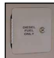
Figure 2-2. Fuel Tank Fill Door
